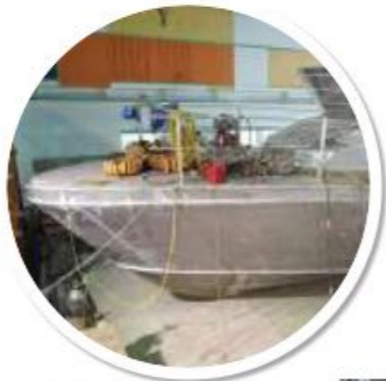
RFV during construction
