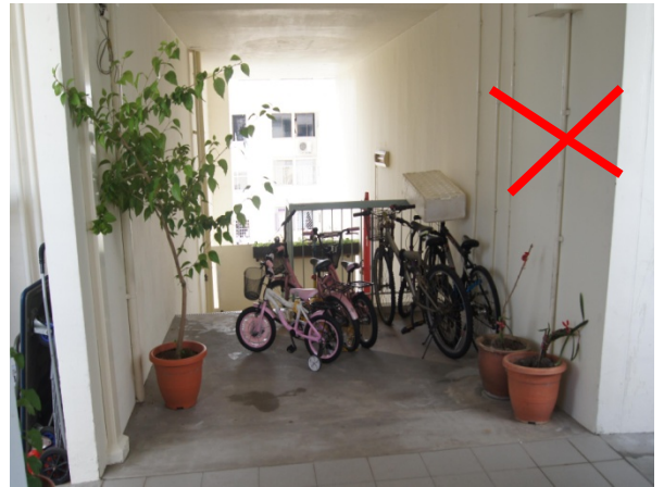
Excessive storage/obstruction at staircase landing
