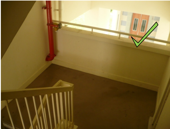
Clear staircase and landing at all times
