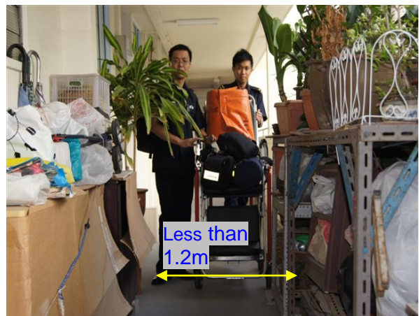
Obstruction to emergency crew access due to constricted corridor
