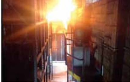
High Bay Storage (Level 4)
