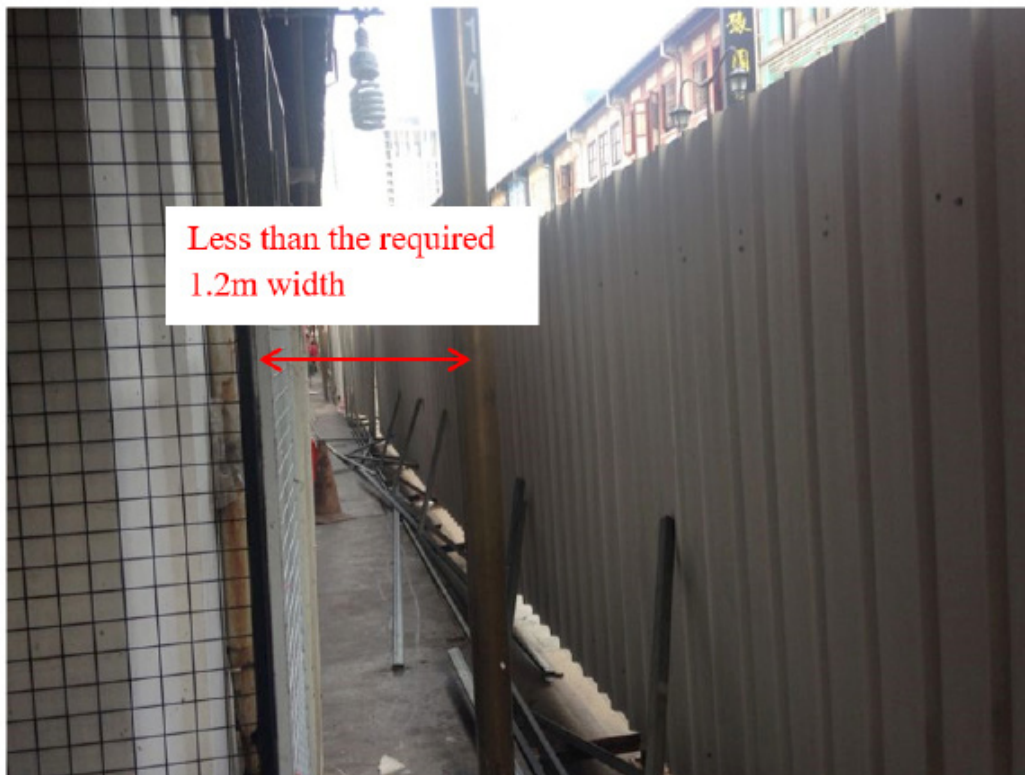
Diagram 9.9.4b.(2) - 1 : Hoarding obstructing means of escape
