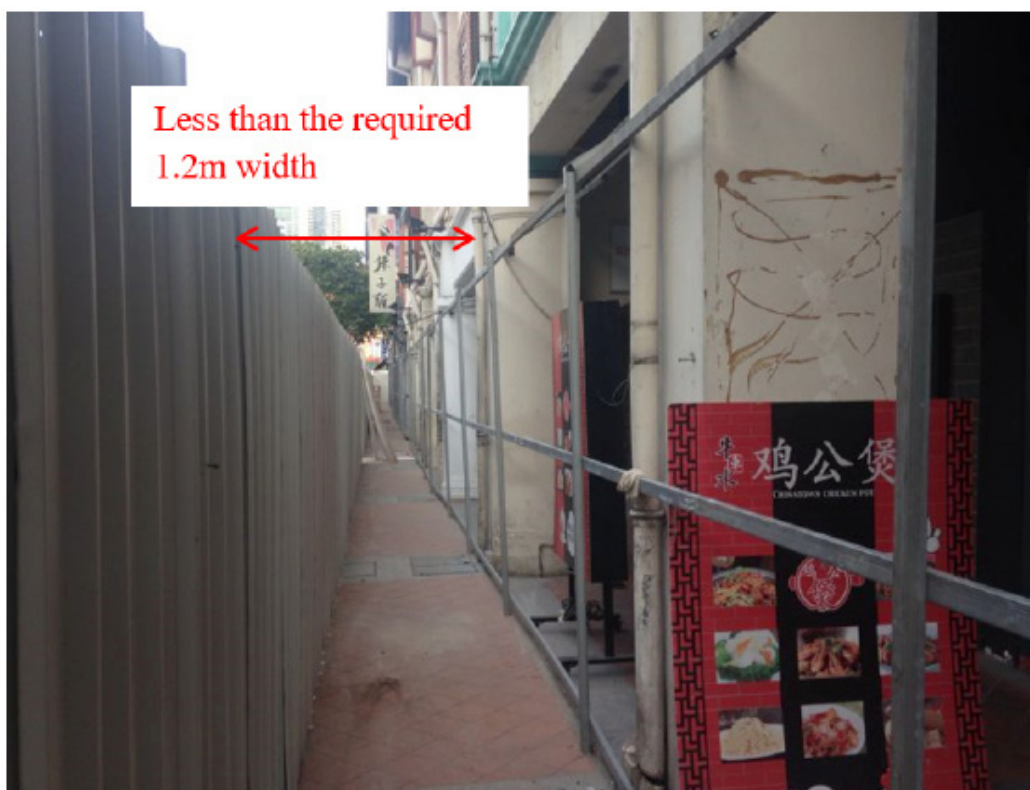
Diagram 9.9.4b.(2) - 2 : Hoarding obstructing means of escape
