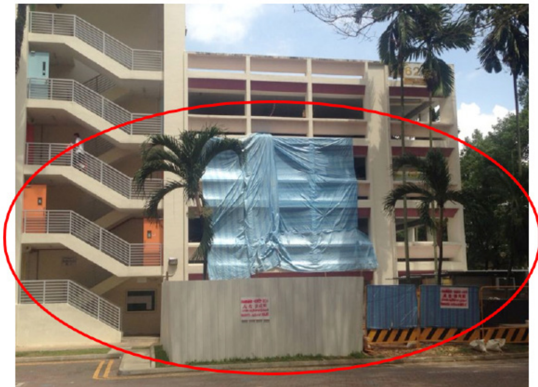
Diagram 9.9.4b.(2) - 4 : Hoarding obstructing openings for smoke dispersal
