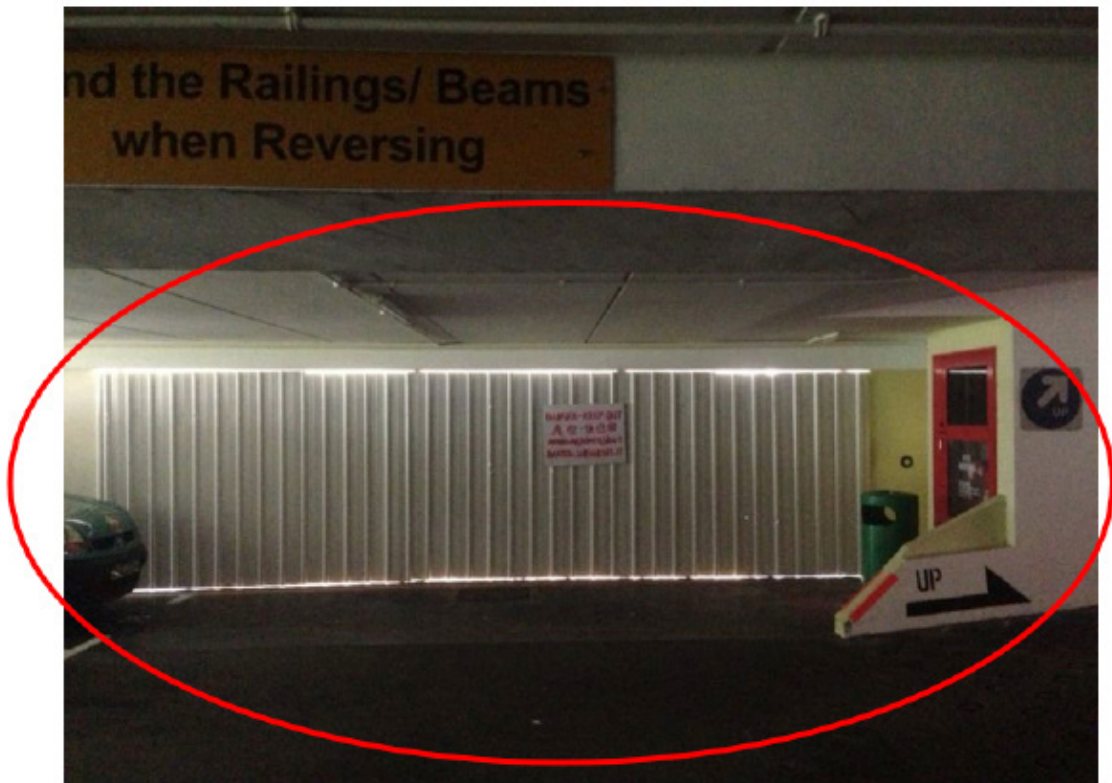
Diagram 9.9.4b.(2) - 3 : Hoarding obstructing openings for smoke dispersal
