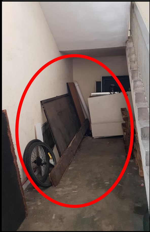
Under Staircase Ramp
