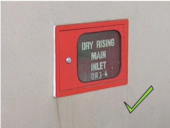
No obstruction to breaching inlet
