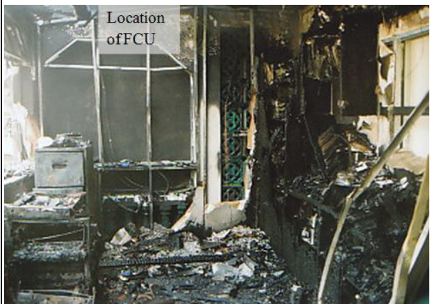
Figure 16. The initial firefighting efforts was unsuccessful and the FCU fire spread to other parts of the office
