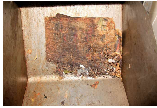
Figure 11. In the refuse hoppers of different levels of the block, burnt marks and partially burnt newspapers were observed
