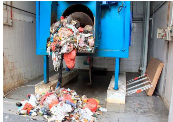
Figure 10. The contents of the Refuse Handling Equipment (RHE) were emptied on each and every occasion of fire
