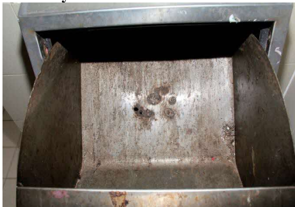
Figure 11. In the refuse hoppers of different levels of the block, burnt marks and partially burnt newspapers were observed
