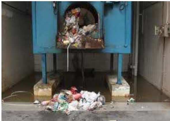
Figure 10. The contents of the Refuse Handling Equipment (RHE) were emptied on each and every occasion of fire
