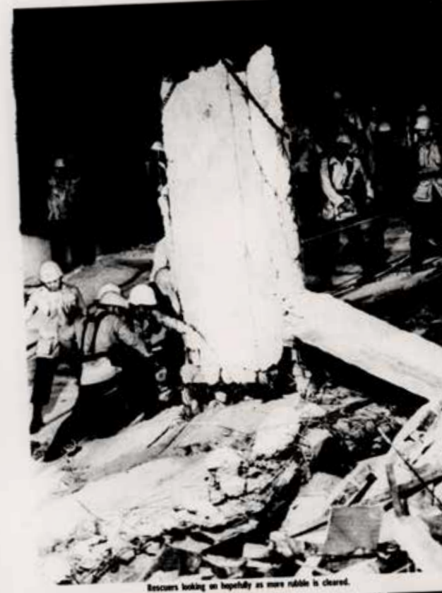
Rescuers looking on hopefully as more rubble is cleared.
