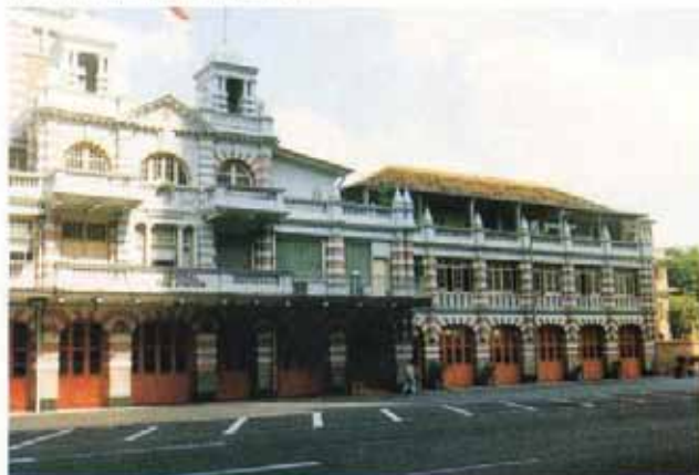
▼ Central Fire Station at Hill Street.
