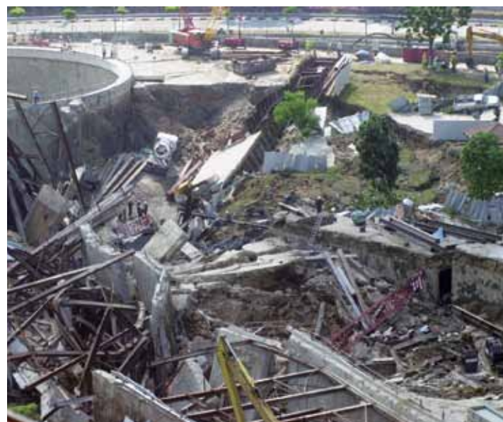
Picture (top left): A view of a collapsed section of the Nicoll Highway.
