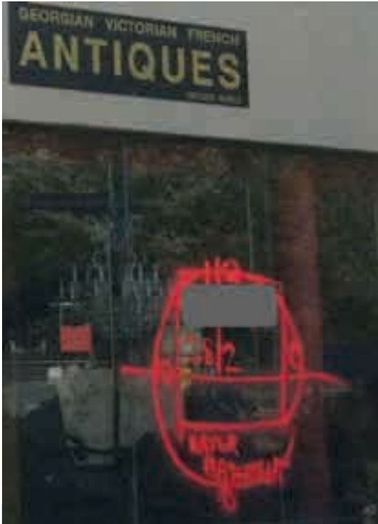
Figure 8 (International Team): Marking that misplaces and abbreviates "No Go". Incorrect placement of "water basement" hazard. Zero fields for victim identification are also applied. Photo by Peter Seager.
