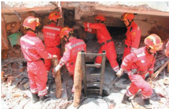
Fig.8 Access and shoring carried out for the second plan
