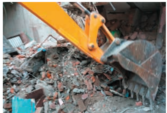
Fig.7 Clearance of the ruins around by excavator
