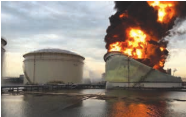
Figure 1: Picture of the JAC Oil Tank Fire
