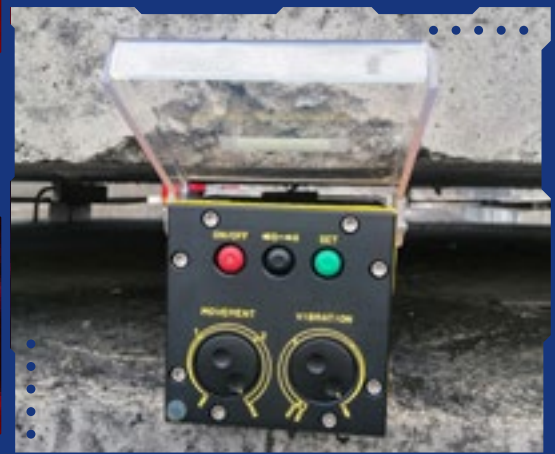
Figure 1: Image of a vibration detector. The detector's alarm would be triggered if the concrete slab moves.
