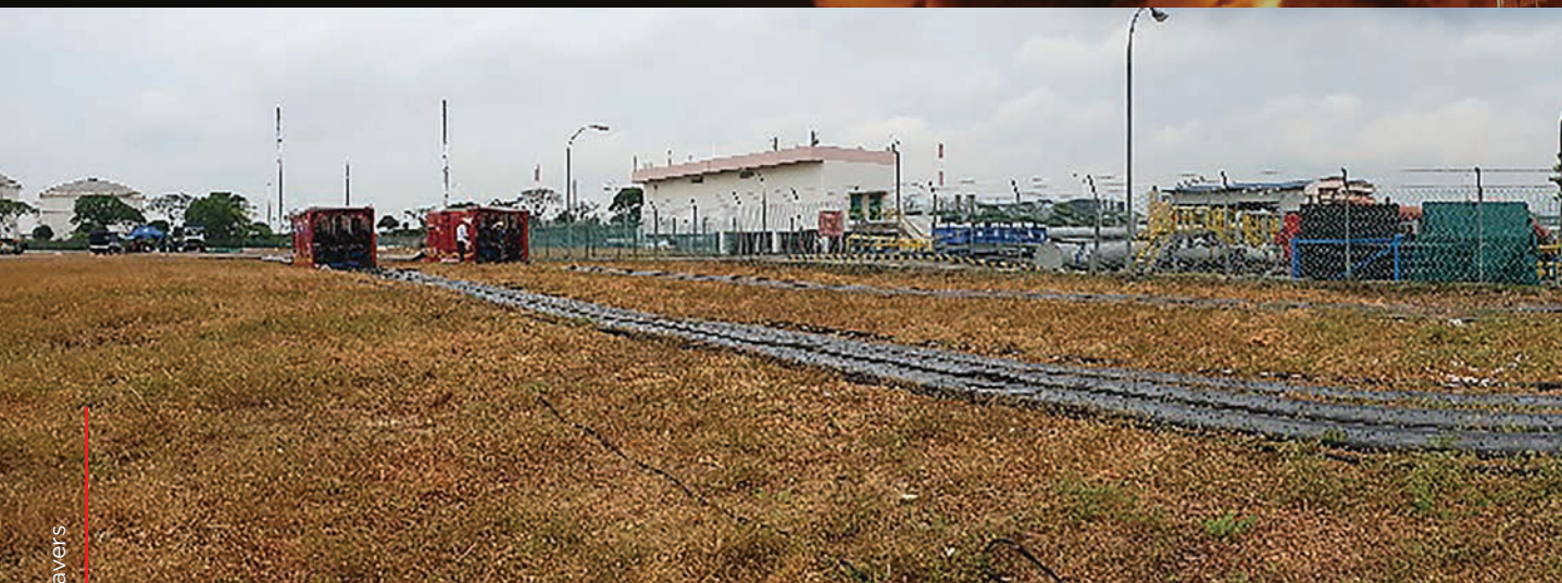
Figure 3: Deployment of submersible pumps from open water source
