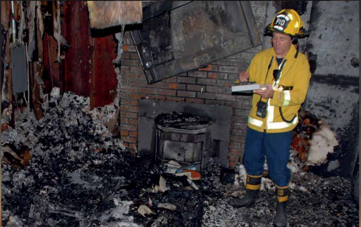
Fire investigators are exposed to toxic chemicals, gases and particulate matter that can cause sickness, disease and even death (Image courtesy of Central Fire Protection District - Santa Cruz County)
