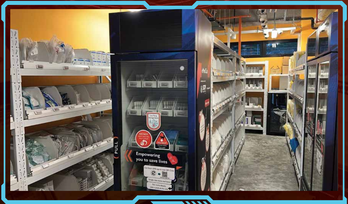
Figure 3: The upgraded AMS featuring shelves with upgraded weight sensors and surveillance cameras
