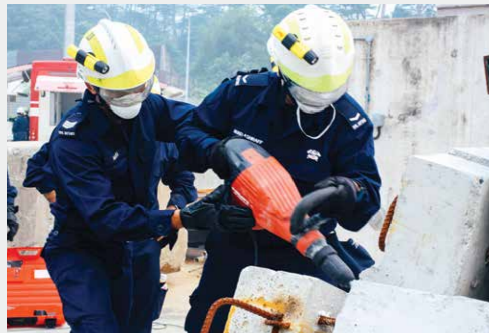
SCDF ORNSmen using a pneumatic breaker during ICT.
