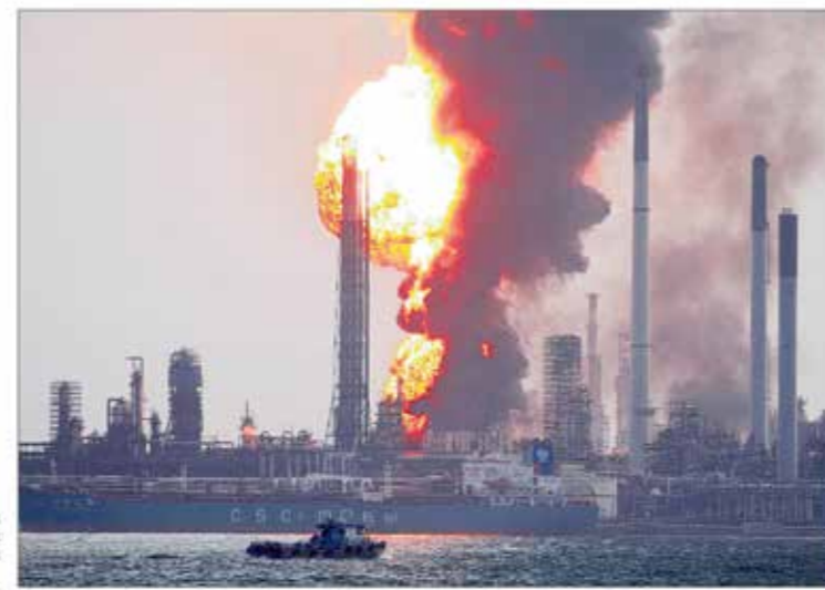
Smoke billows: Plumes of thick smoke and flames seen at Shell's refinery on Pulau Bukom after a fire broke out at 1.15pm yesterday. No fatalities have been reported but one firefighter sustained a minor injury
