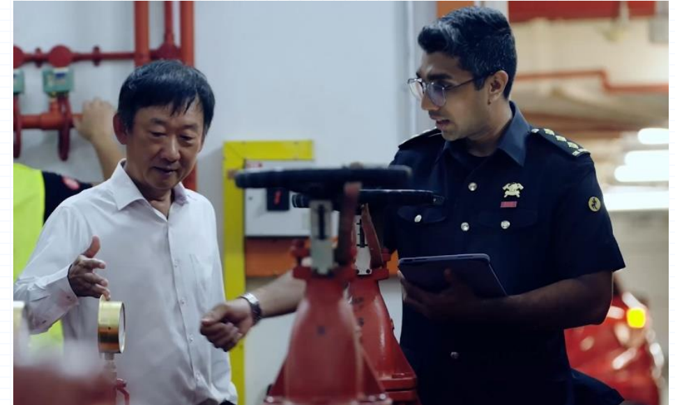
Fig. 1 FSM facilitating SCDF's on-site inspection
