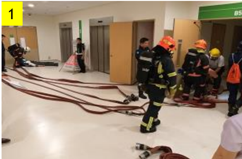
SCDF and CERT members were setting up the dry riser hoses.
